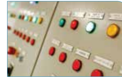
Electric blast panels
